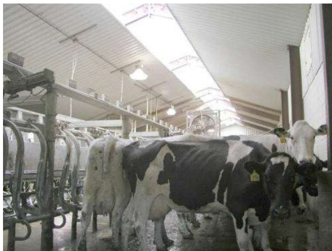
Arntjen ISO lighting/ventilation ridge on top of a milking parlor
